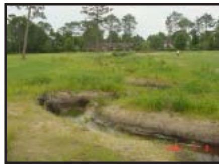
After stream bank restoration.
