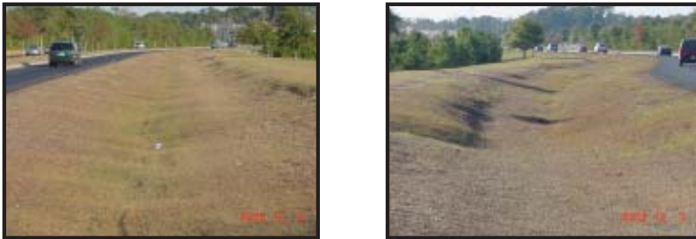
Grassy swales are designed to hold and convey storm water runoff. Swales slow the speed of runoff and allow the water and pollutants to soak into the ground.
