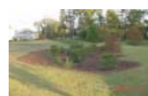
This bioretention area is located in the Storm Water Demonstration Site next to Randall Pond in Wilmington.
